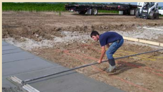
Benjy smoothing concrete during construction of the new facility.
